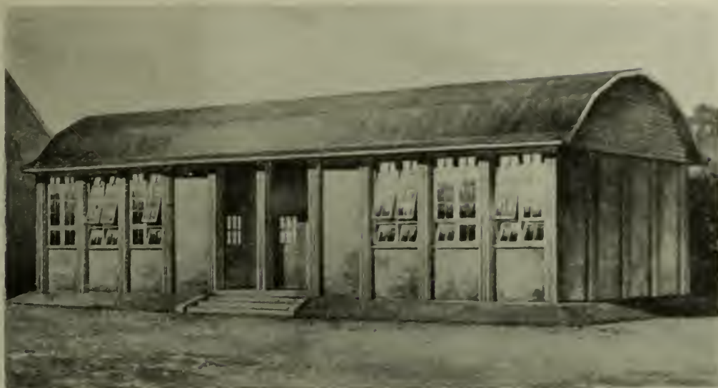
SOMERCOTES BOYS' SCHOOL: EXTENSION. Mr. G. H. WIDDOWS, F.R.I.B.A., School Architect to the Derbyshire County Council.
